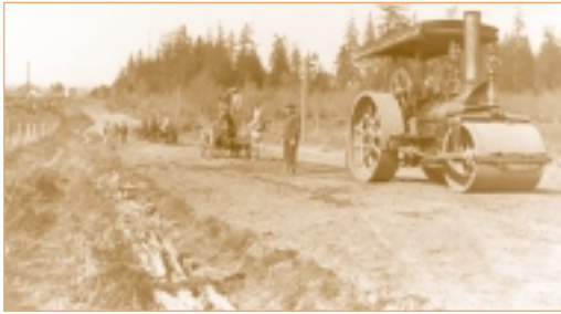
The Boone's Ferry Road was first paved in the early 1900s with gravel from the Nyberg rock quarry. Logs from the old corduroy surface lie in the ditch to the left.
